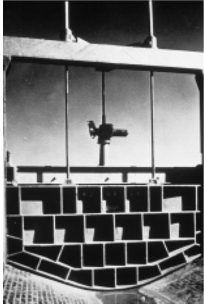
*Above is a Rotork IQ actuator operating a sluice gate. To assure optimum operation, sluice gate stems need to be lubricated regularly.*
