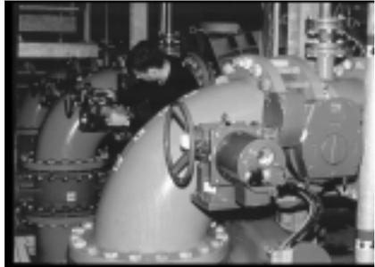
*Pictured above are Rotork IQ actuators on butterfly valves.*
